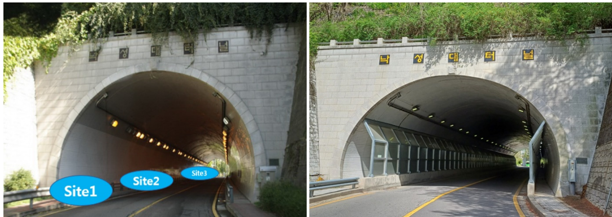
Figure 1. The places where measurement was conducted. Left is before the safety walls were installed and right is after installation
