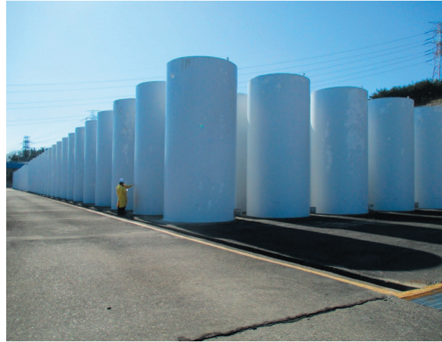
Fig. 1. Silo dry storage facility at Wolsong NPP site.
