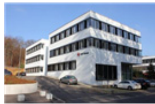
Fig. 7. 2 nd Research Building
