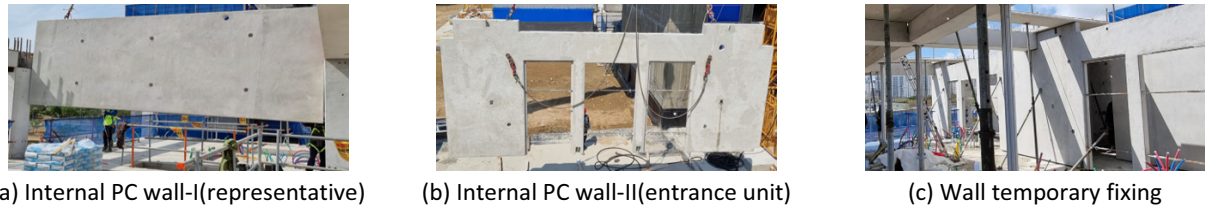
Figure 5. Internal PC wall erection and detail
