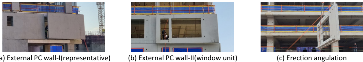
Figure 6. External PC wall erection and detail
