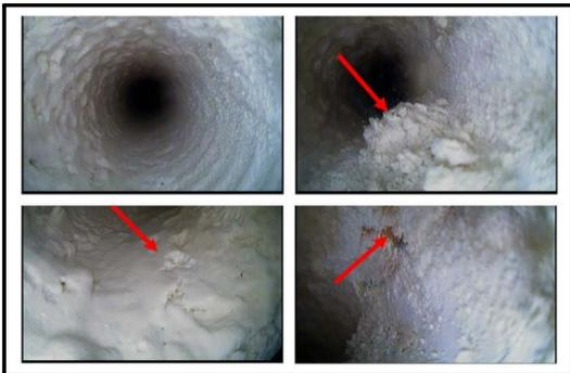
**Fig. 1.** Sedimentary dust in dry scrubber inlet piping.
