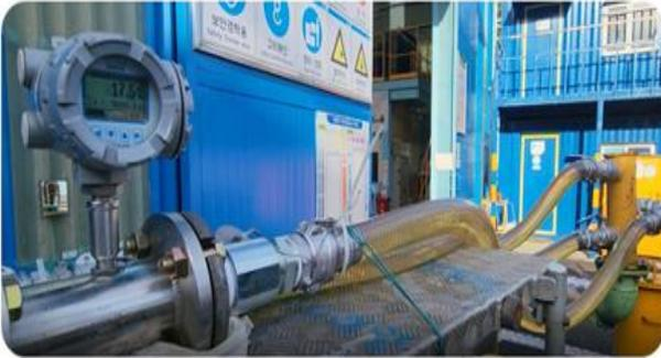
Fig. 11. Flow meter and transparent hose to Oil Return.
