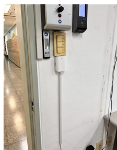
Fig. 6. Entrance side installation
