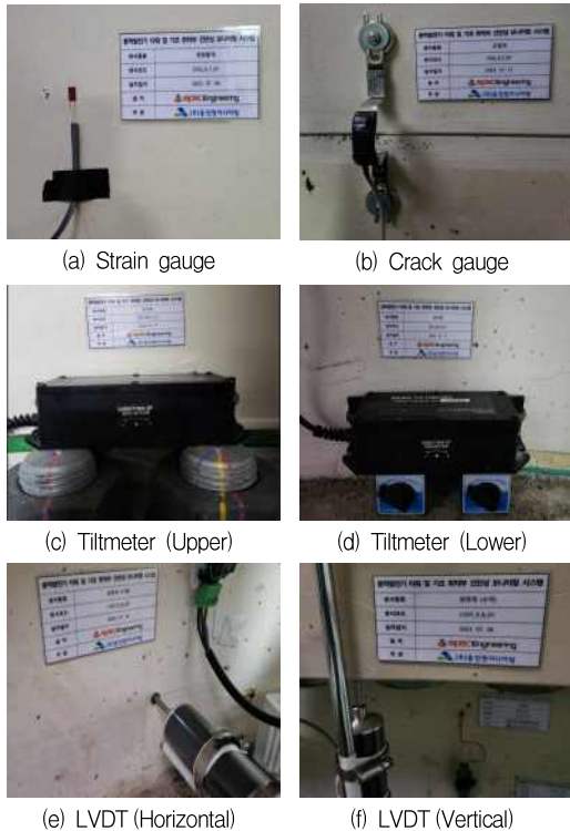
Fig. 9 Photos of installed sensors
