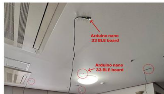
Fig. 2. Attach five boards to the ceiling
