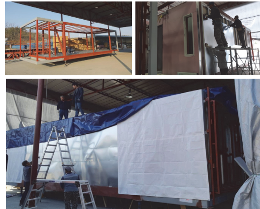
Fig. 1 Prefabrication of modular
