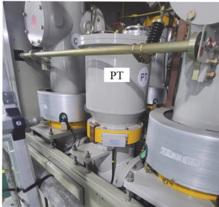
Fig. 1. Application of tank type PT in GIS.
