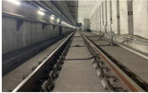
(a) Tunnel section concrete track
