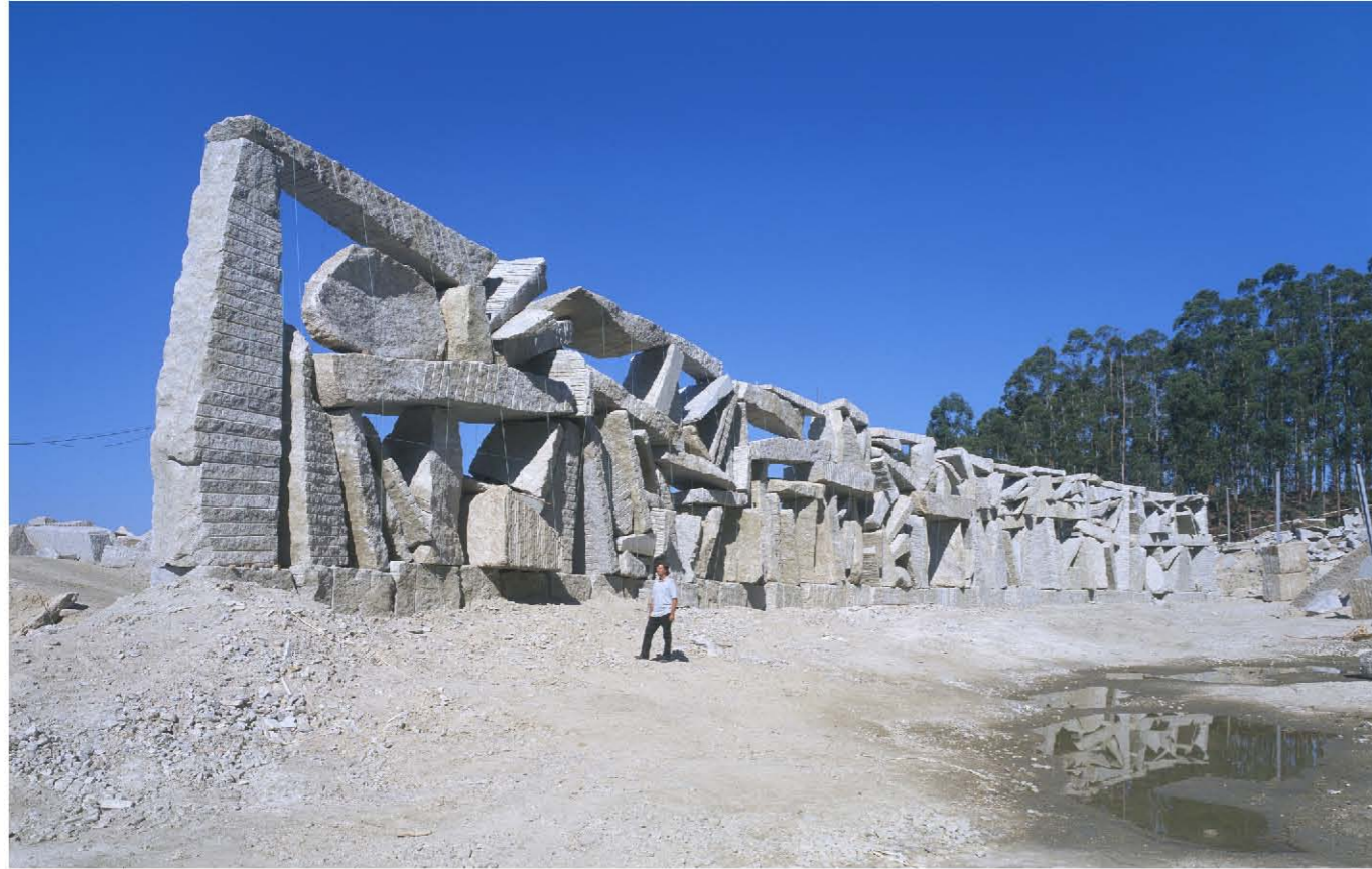
SGAE Headquarters, Santiago de Compostela, Spain, 2007 / Ensemble Studio
