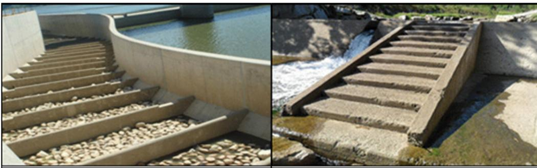
Fig. 1. Standard (left) and non-standard (right) of stepped fishway (KRC, 2023)
