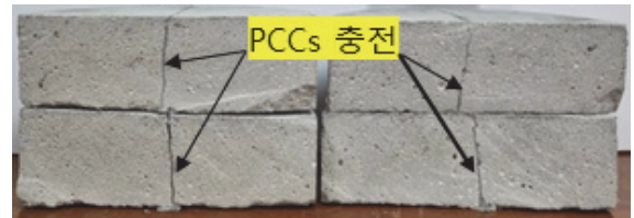
Filled PCCs in Crack
