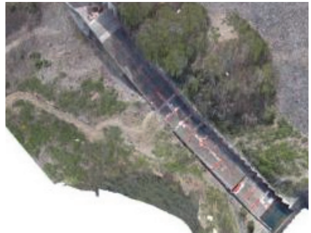
Fig. 10 3D Digitalized Safety Inspection Map of JAR Dam Spillway
