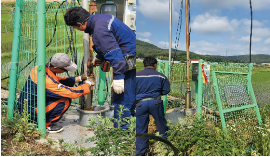
Fig. 1. Observation hole construction.
