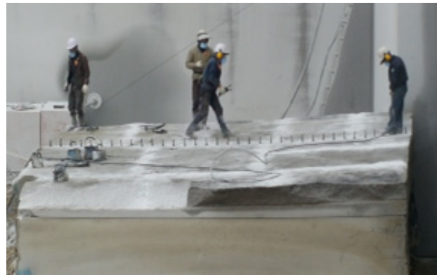
b. Rock chipping workers
