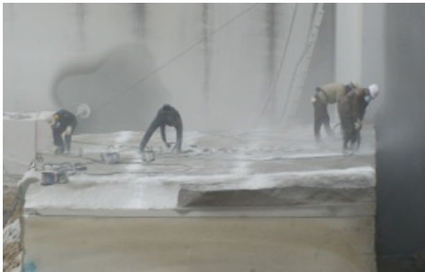
a. Rock chipping
