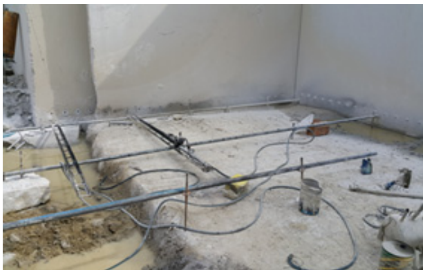
c. Horizontal rock drilling
