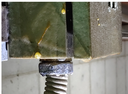
Fig. 1. Condensation in underground utility tunnel
