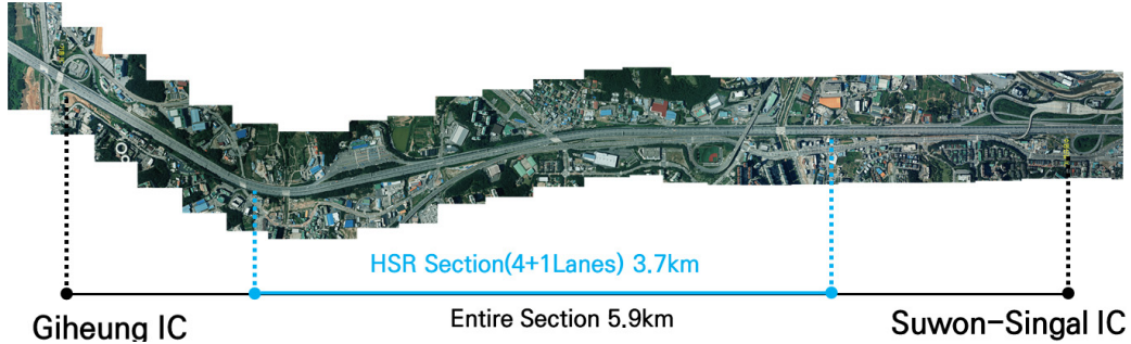
<Fig. 2> Target expressway segment for analysis(Giheung IC - Suwonsingal IC)
