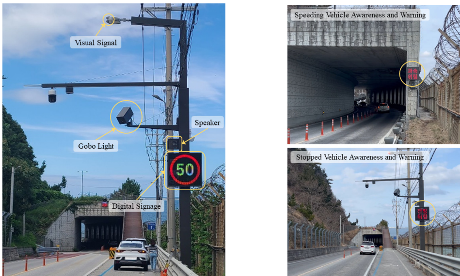
<Fig. 1> Display devices of smart road lighting platform <Fig. 2> Examples of traffic safety information service
