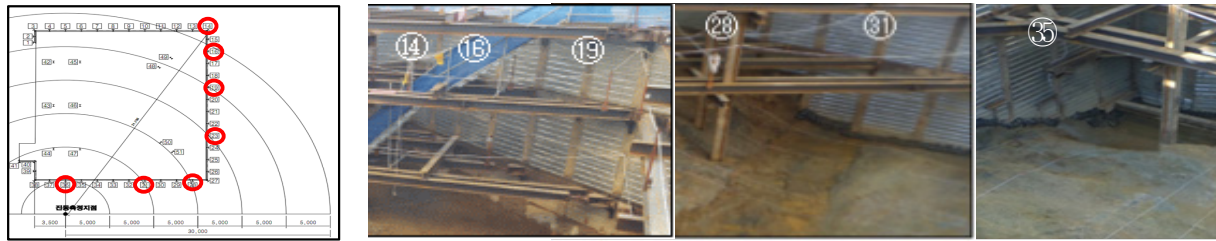
Fig. 3. Vibration Measuring Point and Earth Retaining Picture
