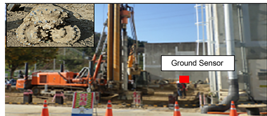
Fig. 2. Tricone-Bits Machine & Sensor Location
