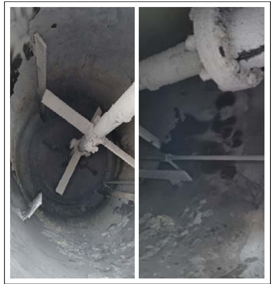
Fig. 5. Inside the wrecked reactor.
