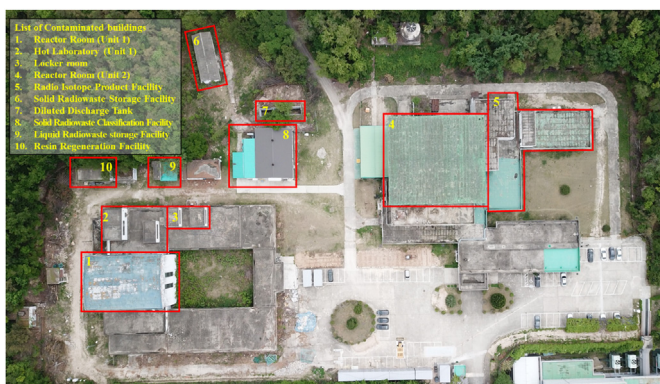
Fig. 1. Location map of contaminated buildings at KRR-1&2.
