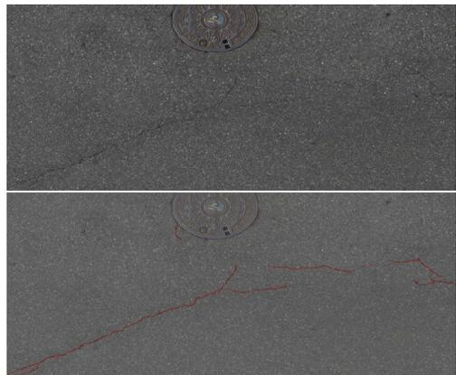
Fig. 13. Image data (Above: Original Image, Below: Crack Detection Result)
