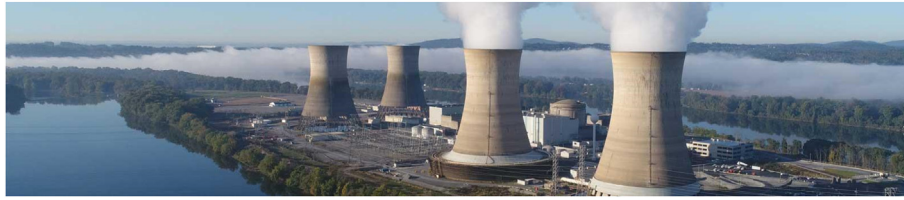
Fig. 1. Three Mile Island Generating Station Unit 1, which permanently closed on September 20, 2019.
