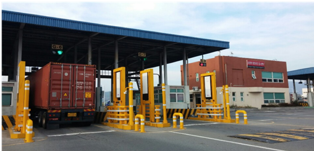
Fig. 2. Radiation portal monitor at a Korean airport.
