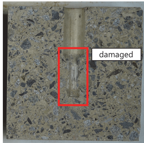
Fig. 9 Bond-slip destruction pattern: Type 2
