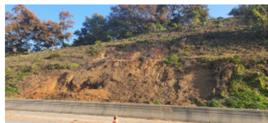
Fig. 1. Slope surface failure and erosion
