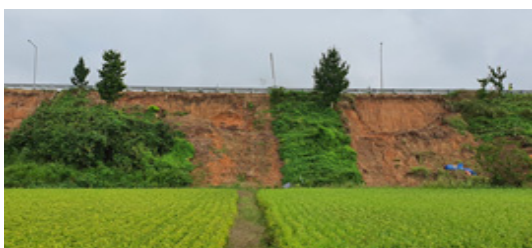
Fig. 1. Slope surface failure and erosion
