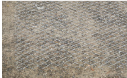
(b) High-strength net (thickness 3.2mm, 1,000MPa)
