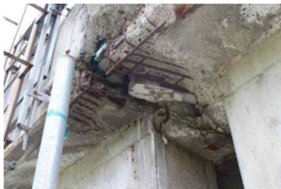
(a) Deck Slab End
