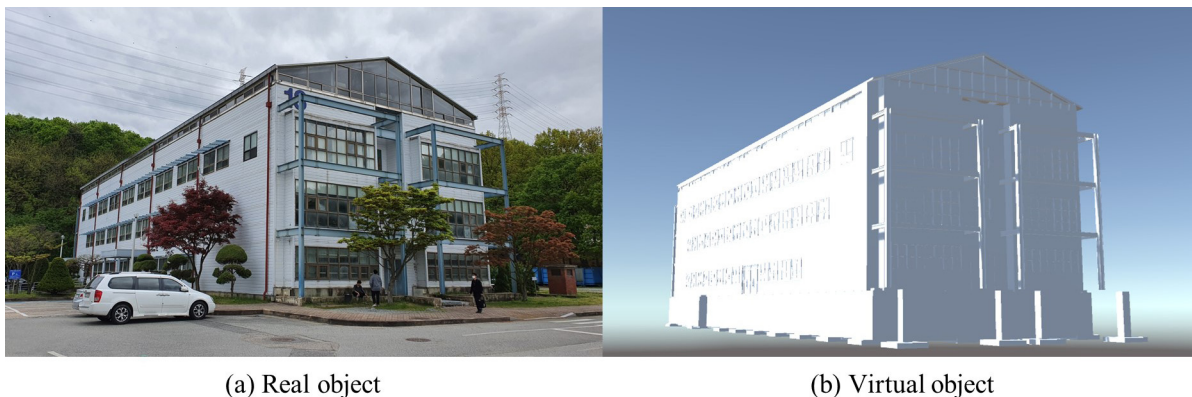
Figure 5. Real target object structure and its 3D shape model in virtual space
