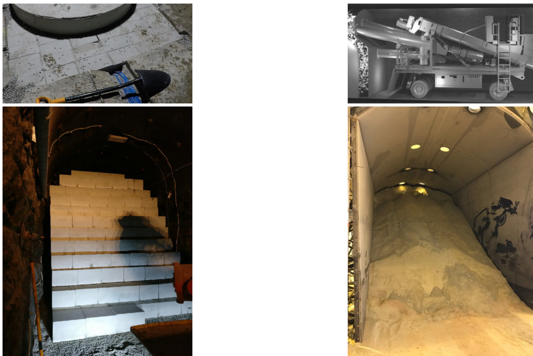
Fig. 5. Backfilling solutions of block/pellet (left) and granular (right) types in the full-scale in-situ system test (Johanna and Ville, 2022)
