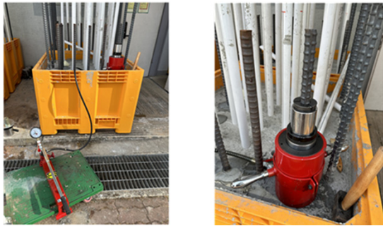
(a) Pullout capacity test of 25 mm deformed bar
