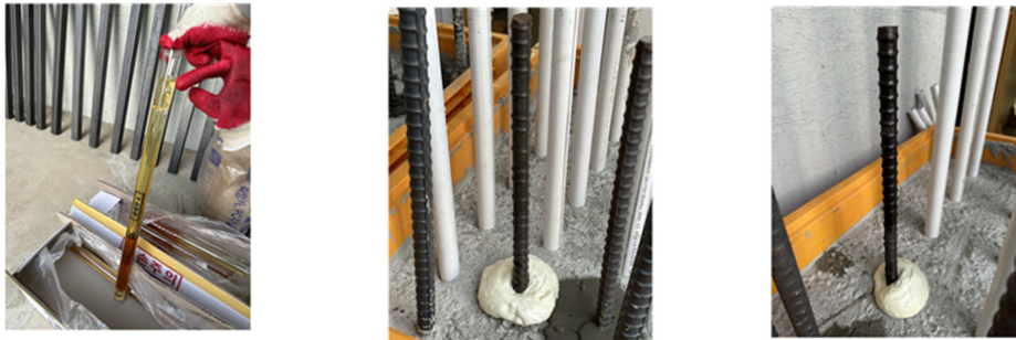
(b) Installation of deformed rebar after inserting the resin tube into a drill hole
