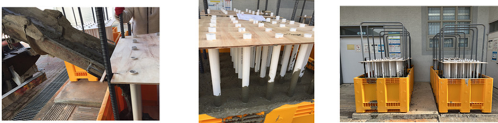
(b) Concrete pouring for making
