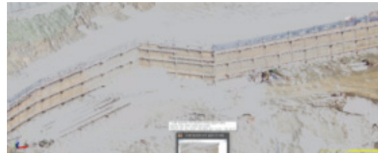
Fig. 7 Retaining wall sections verified with MMS pointcloud data
