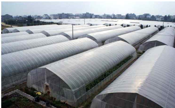
FIGURE 1. Examples of the greenhouses with plastic covers and arched roofs in South Korea (a figure captured from http://www.newsfarm.co.kr/news/articleView.html?idxno=49997 )
