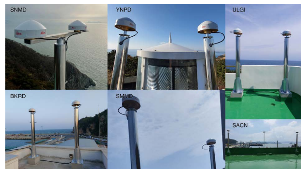
Fig. 4. Installed GNSS antennas at POINT reference stations: SNMD (top left), YNPD (top middle), ULGI (top right), BKRD (bottom left), SMMD (bottom middle), and SACN (bottom right).
