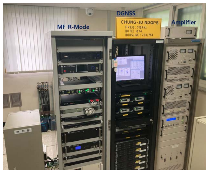
Fig. 5. MF R-Mode transmitting system installation of Chungju.
