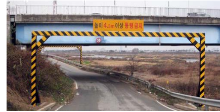
Fig. 7. Height limit clearance.
