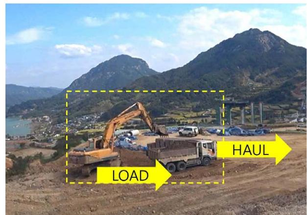
Fig. 2. Process analysis for earthmoving operation (example)
