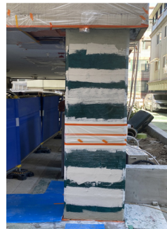
(b) Retrofit Method of Fiber Sheet
