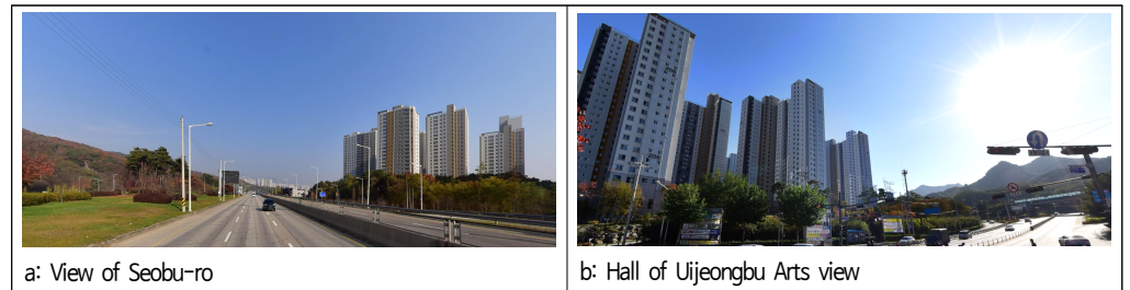
Figure 2. View of Seobu-ro (L: Jikdong Neighborhood Park, R: non-park facility apartment complex) and hall of Uijeongbu Arts view (L: non-park facility apartment complex, R: Jikdong Neighborhood Park Sapae mountain)
