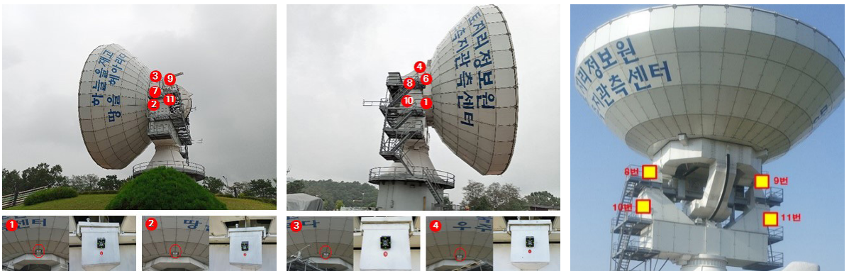
Fig. 1. Location of targets on VLBI antenna (NGII, 2019)
