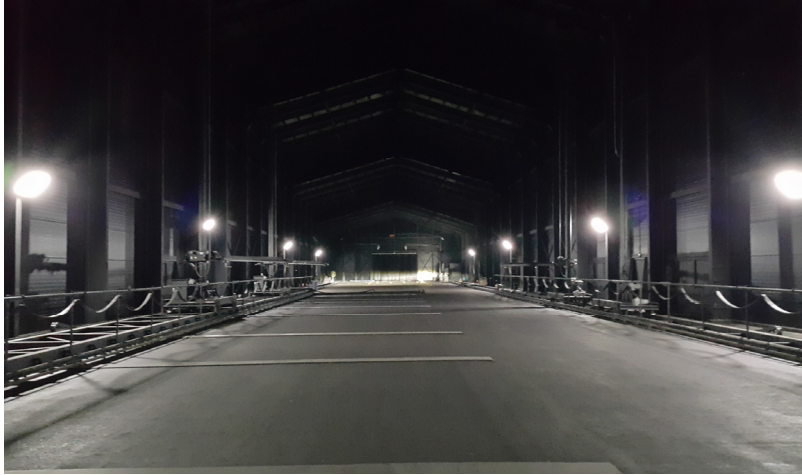
<Fig. 1> Testbed to demonstrate lighting performance(KOPTI)
