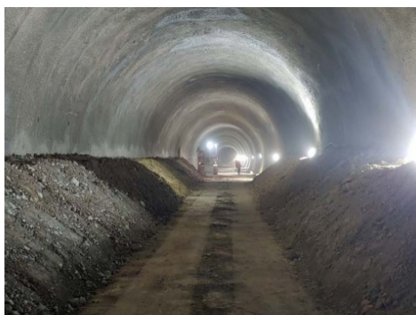
Fig. 6. Preloading of the research tunnel wall
