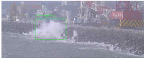
(a) Correct overtopping detection
