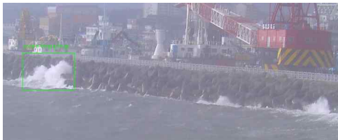
(b) Incorrect overtopping detection
