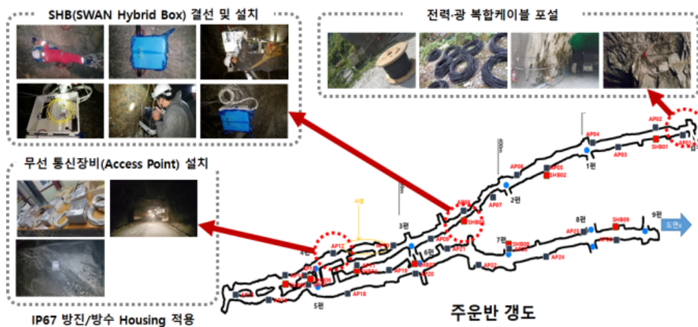
Fig. 11. Installation of communication equipment in the mine
