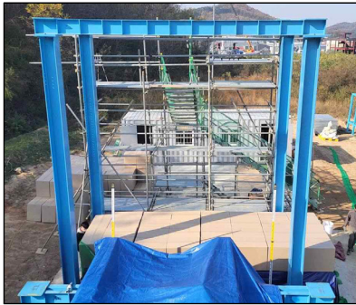
Fig. 7 Main Test Fixture for Ground Separation Test
