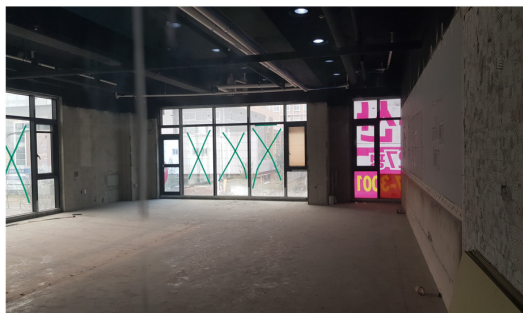
(c) Water leakage due to poor facility management
