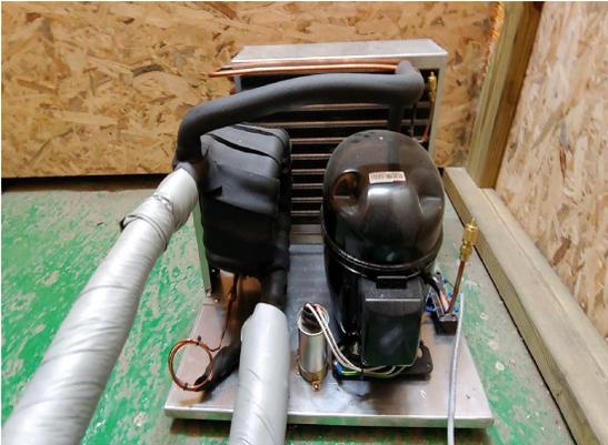
Fig. 4 Chiller installed inside a mobile modular house
