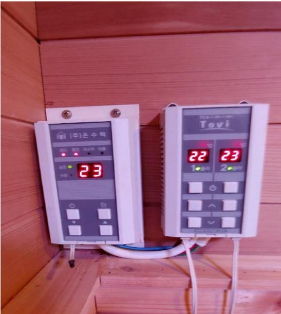
Fig. 5 Air temperature controller and temperature sensors inside a mobile modular house
